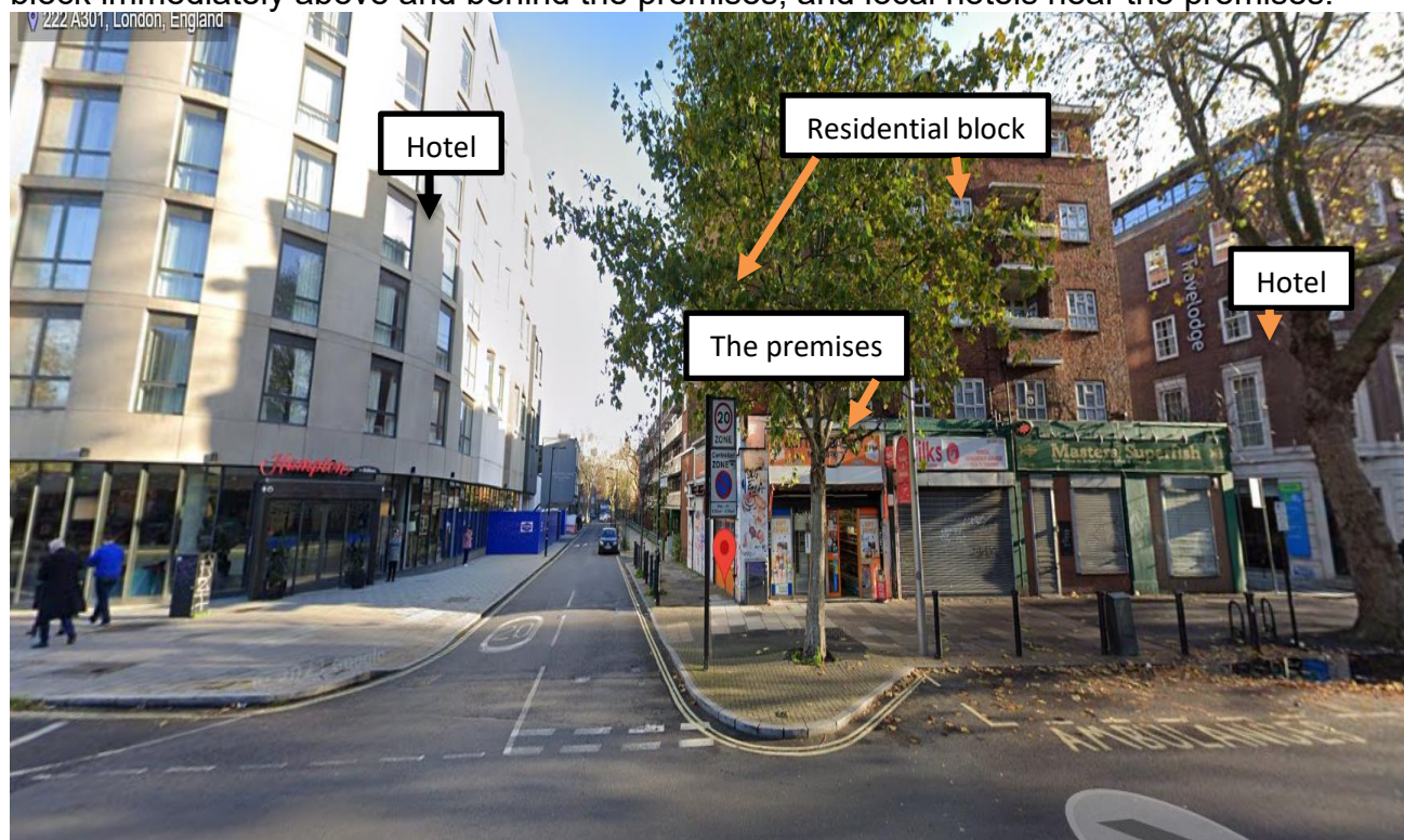
Figure 1: View looking north east across Waterloo Road showing the premises, housing block immediately above and behind the premises, and local hotels near the premises.
